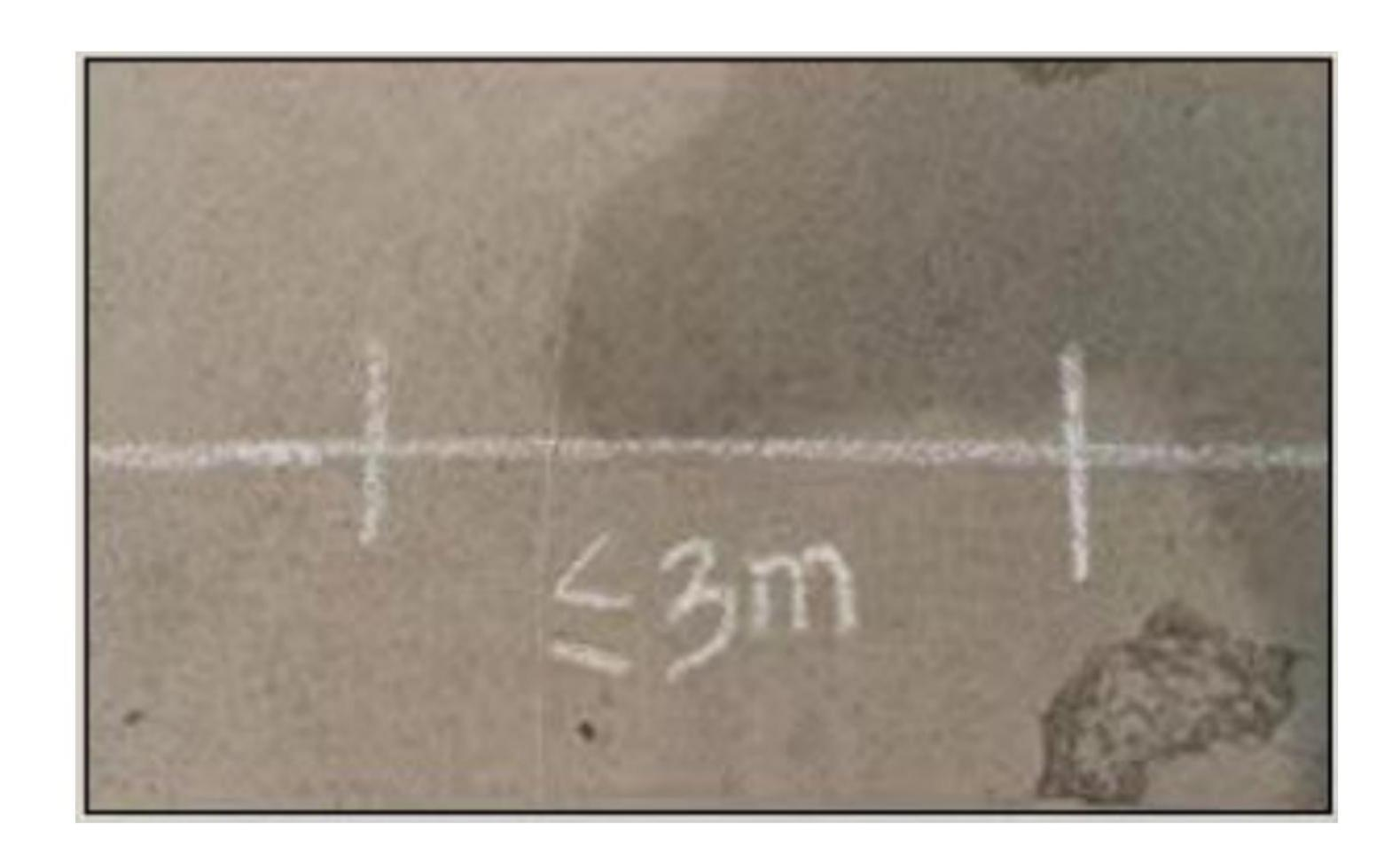
Step 1: Mark the proper installation position. Normally,3m distance between road studs will be better.
