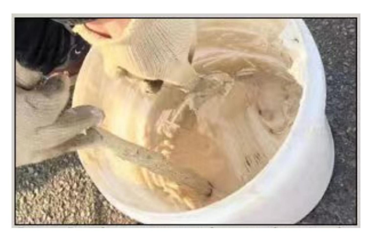
Step 3: The epoxy glue ratio: A glue and B glue is 1:1. The glue should be mix well-distribute with the electric drill, 40-50g will be used for each stud.
