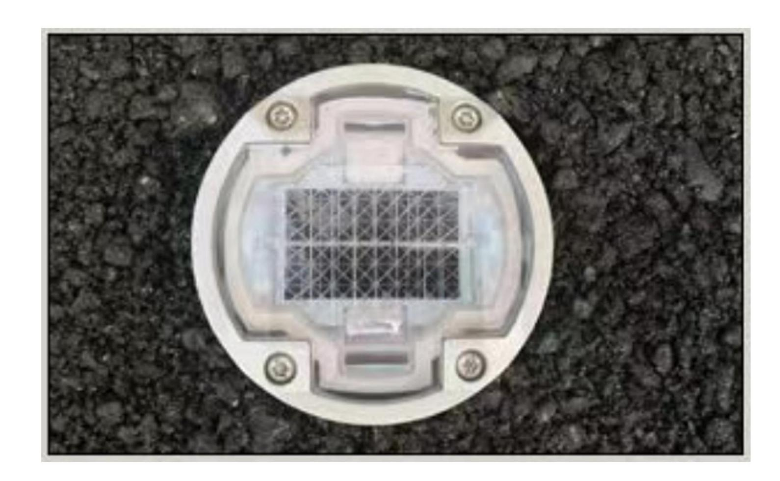
Step 5: Use the knife to clean the surrounding overflow glue after the installation and remover all debris form the carriageway.
