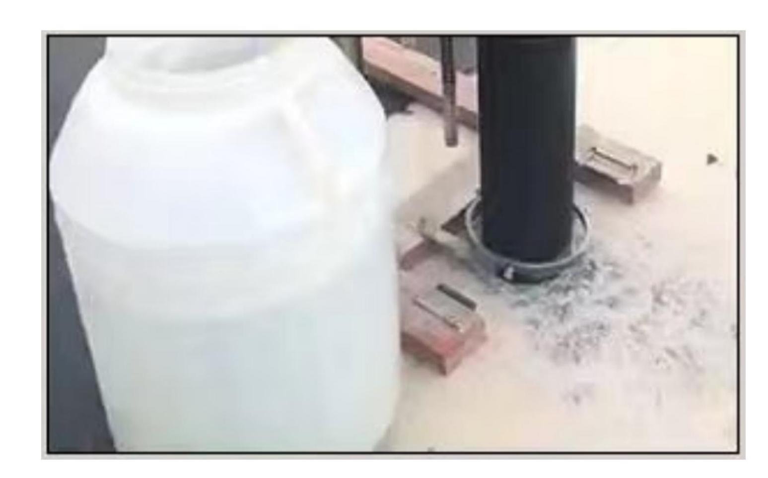
Step 2: Use the core drilling machine to drill a hole according to the actual size of the shank. Dry the holes with a blowtorch and clean the hole.
